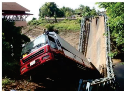
Figure 2.9. Bailey bridge collapse due to deterioration (Chowdhury, N.d.)
