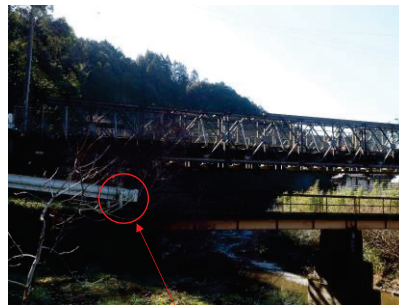
(b) Determination of a deflection based on the relationship of the target and fixed guard rail bolt - Plane view.
