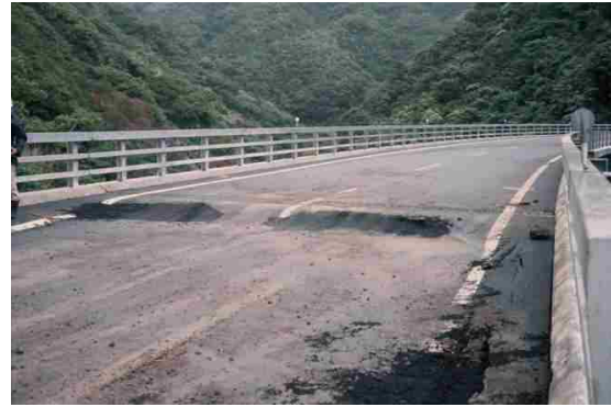
図-3.5 橋台裏込め部の沈下
