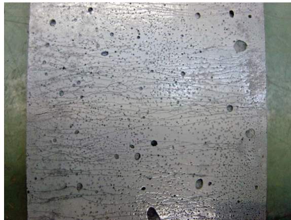
写真-2.1 ひび割れ分散性状 [3]
