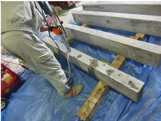
(c) 圧入孔の削孔
