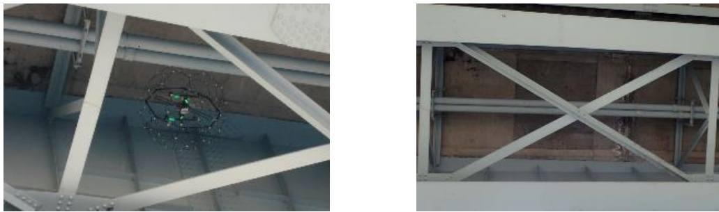
Figure 4.7 Narrow space in steel girder by attachments
