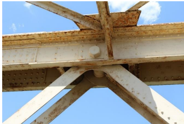
Figure 4.10 Panel point of the truss bridge
