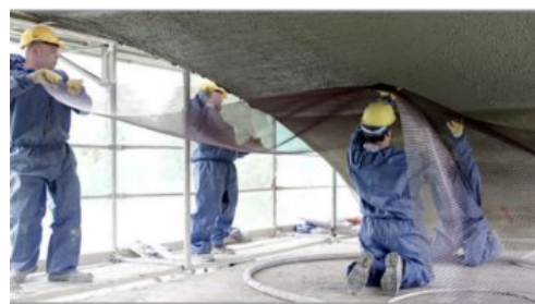
d) Strengthening by TRC (Naila, Germany)
