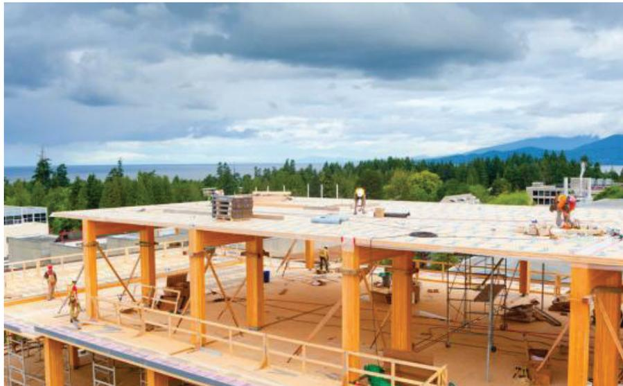
**Fig. 1.1.6 CLT timber building 5**
