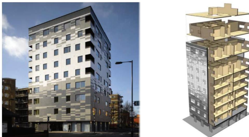
**Fig. 1.1.2 CLT timber building 1**
