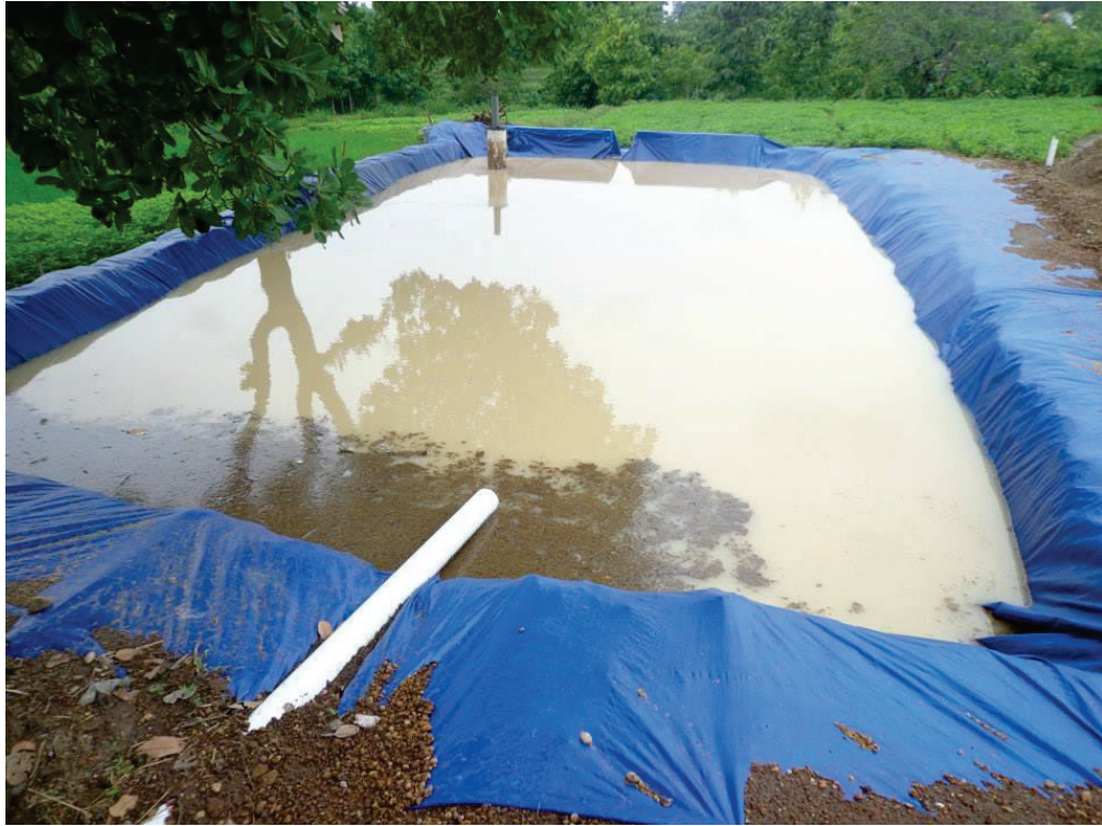
Figure 2.4 SFR1 was constructed under cashew canopy
