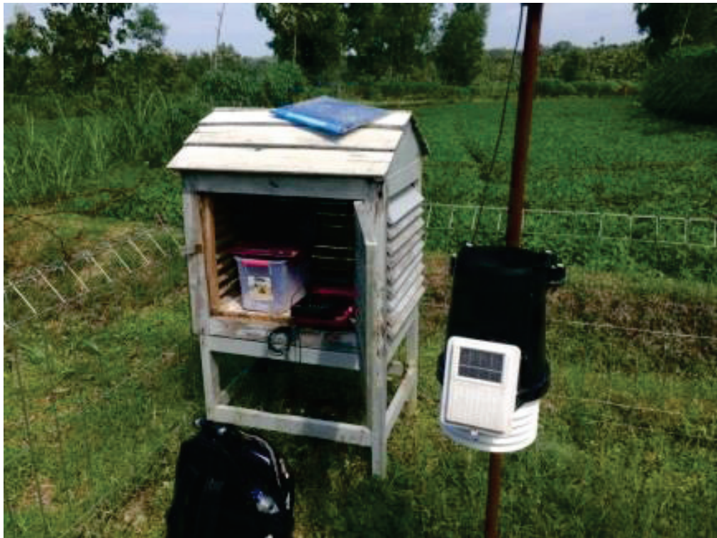
Figure 2.9 Automatic Water Station was installed near SFR2
