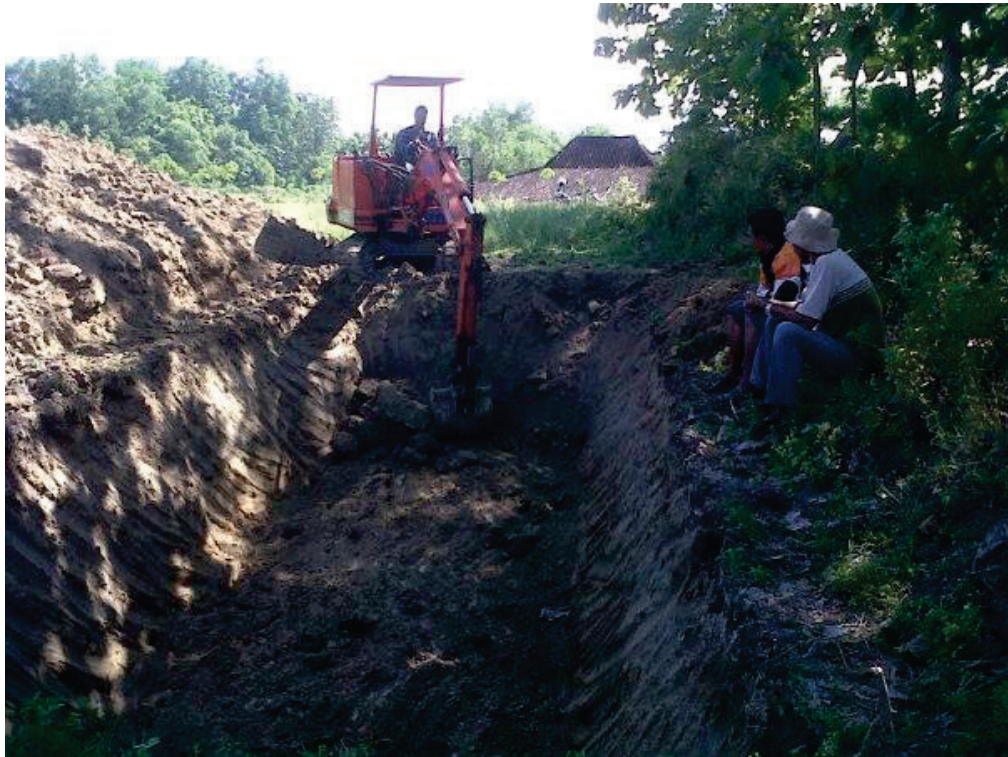
Figure 2.2 SFR2 was constructed by Backhoe
