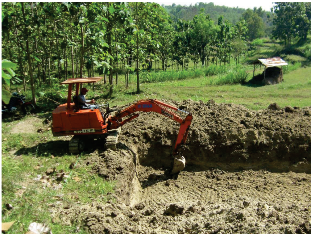
Figure 2.3 SFR3 was constructed by Backhoe
