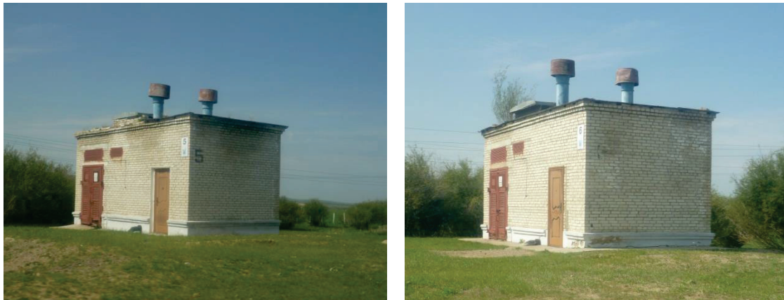
Figure 3.4 Photo of deep-wells
