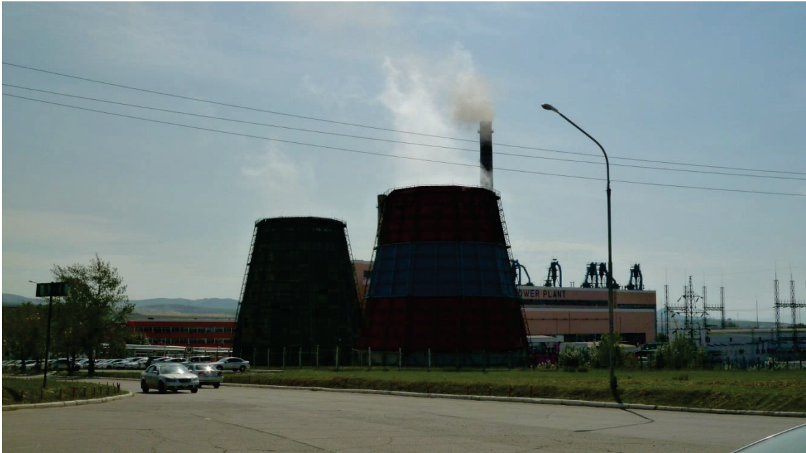
Figure 3.28 Photo of thermal power station of the Darkhan City
