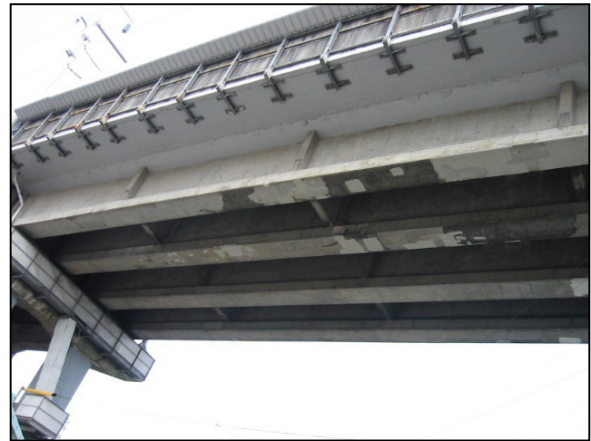
写真-8 橋梁PC桁
